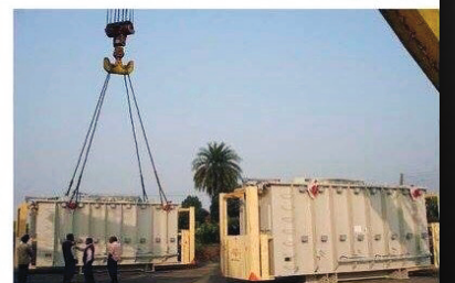
Unloading of 80 M.Ton heavy transformer at river jetty
